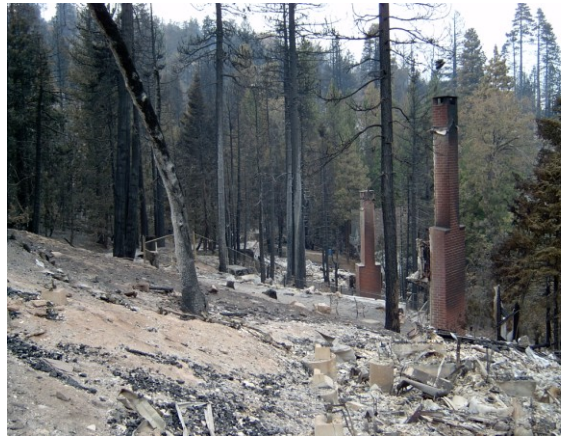
Figure 2. Unconsumed vegetation surrounding destroyed homes indicates ignitions from lower intensity surface fires and/or firebrands directly igniting homes. These homes were among hundreds of homes simultaneously exposed to ignition and unable to be protected. The wood construction burned to total consumption.
