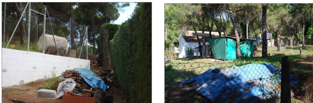
Figure 3. Bad maintenance of property structure's borders and accumulation of many types of fuels. Source: Quesada 2011.
